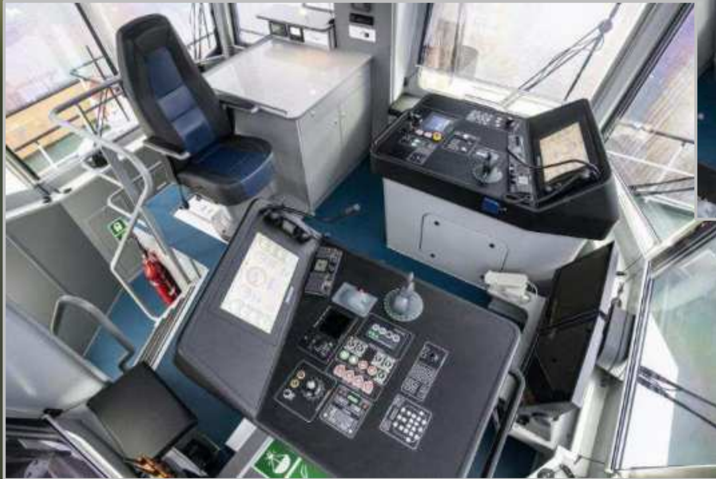
Triac builds these console sets for Damen Shipyards.
