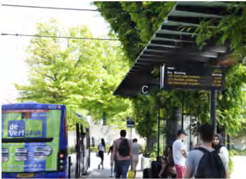
Installation Site: Netherlands
