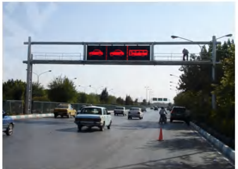
Installation Site: Iran
