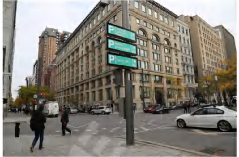
Installation Site: Canada
