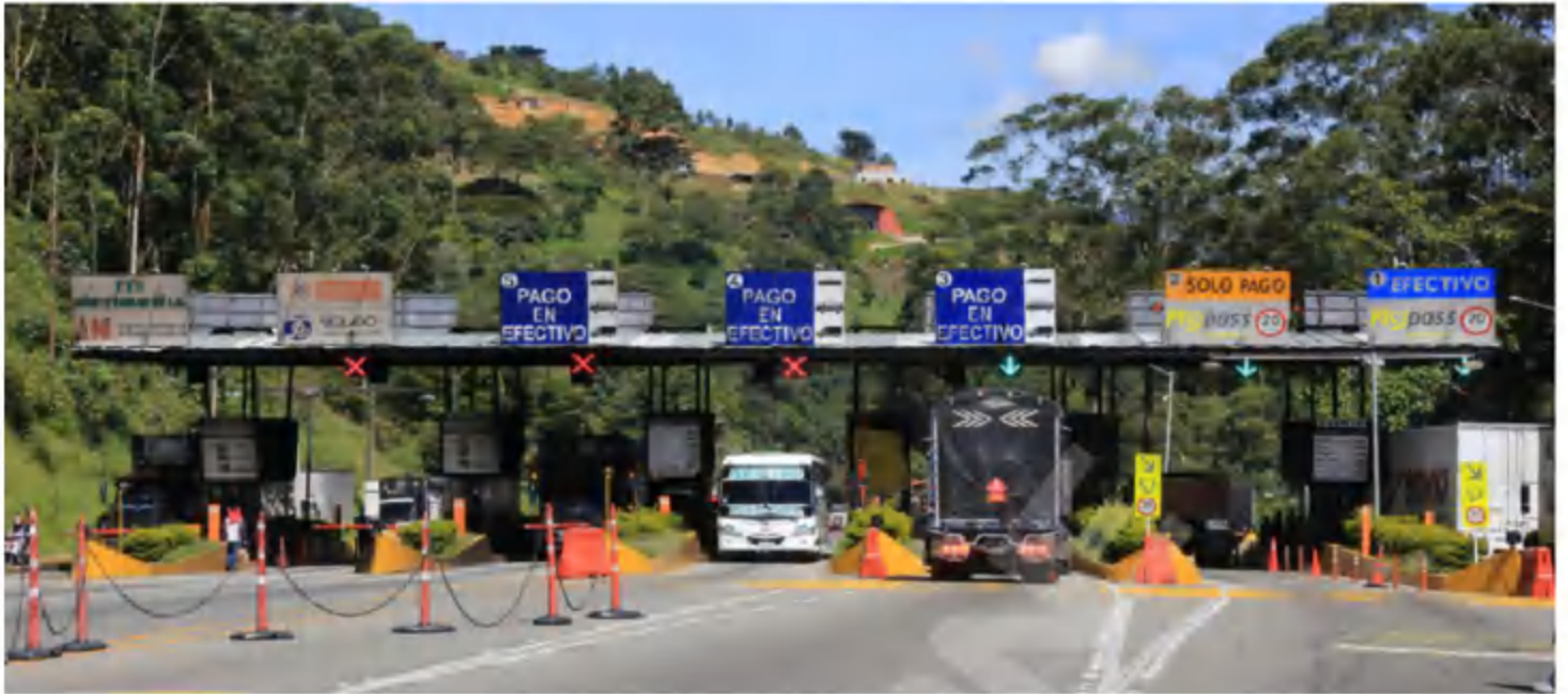
Installation Site: Colombia
