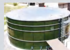
Trough Deck Roof
