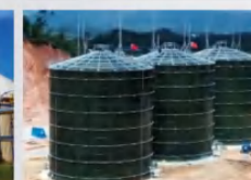
Tapered Steel Roof
