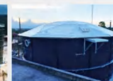
Geodesic Dome Roof
