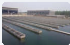
Municipal drinking water plants
