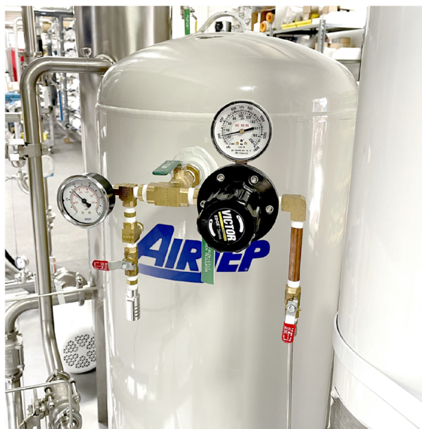
Oxygen Generator Accumulation Tank
