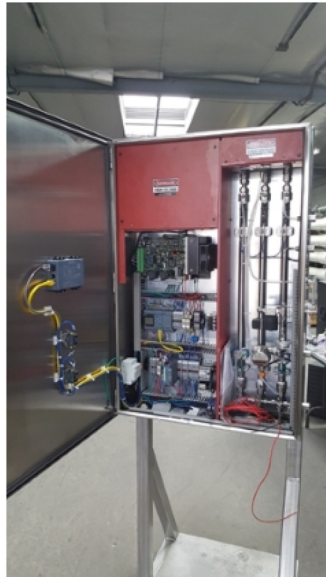
Sample Interior of Ozone System Cabinet
