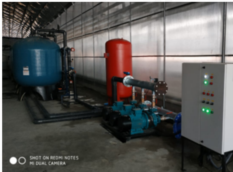
40 - 60 m 3 /h Sand-Carbon System - 72 m 3 /h Reverse Osmosis System
