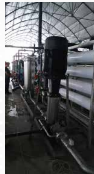
40 - 60 m 3 /h Sand-Carbon System - 72 m 3 /h Reverse Osmosis System
