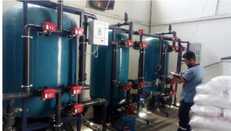
20 - 25 m 3 /h Sand - Arsenic Carbon Dublex Softener System
