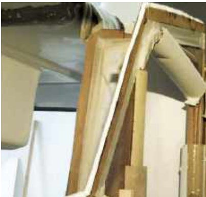
Fig. 11 Sikaflex®-292i applied to a lightweight panel prior to fitting
