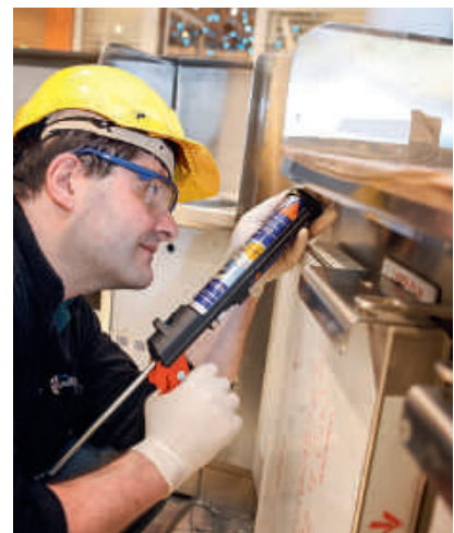
Fig. 9 Application of Sikaflex®-291i
