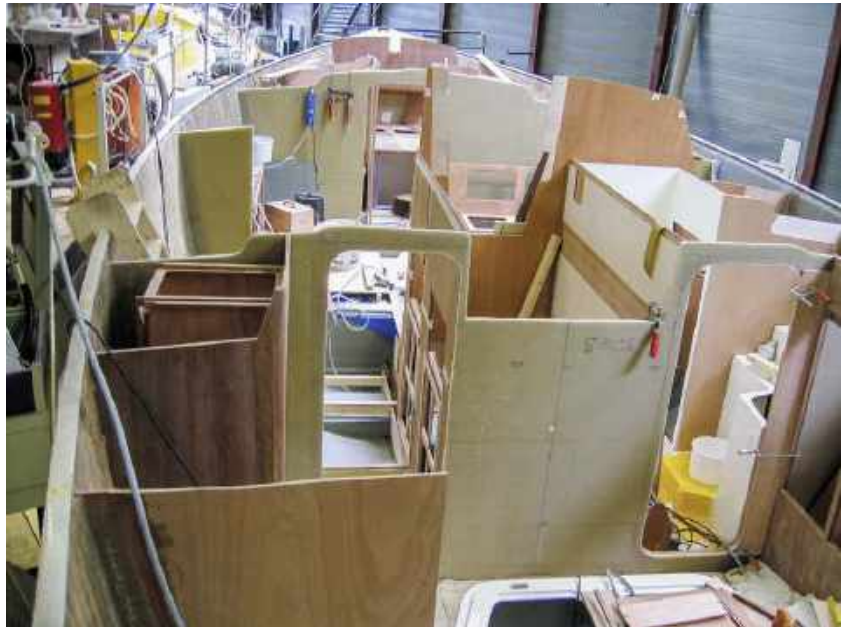
Fig. 12 Lightweight panels being fitted to an open hull
