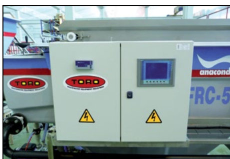
Dynamic graphic cabinet: PLC touch screen, alarm history, status, hour meter...
