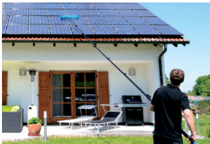
Cleaning from the ground with telescopic-lance
