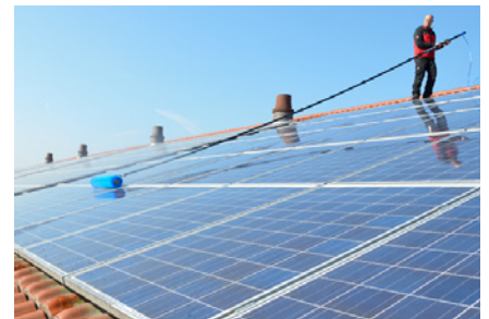
Cleaning from the rooftop with telescopic-lance
