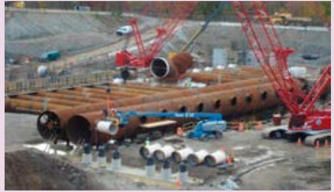
▲ Building the water purification plant for New York City.
