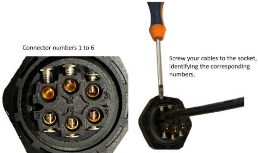
Figure 9: Installation of the 6 cables on the bulkhead connector
