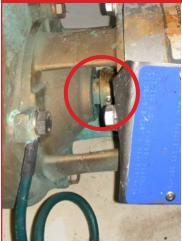
Traditional direct-drive pumps leak at the shaft seal causing them to fail.
