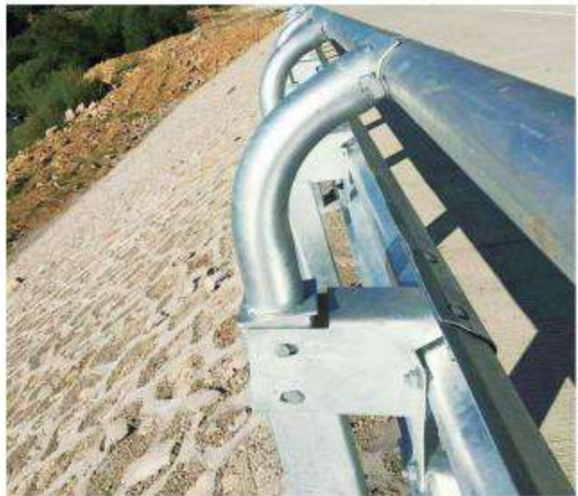
● GUARDRAIL END TERMINALS
