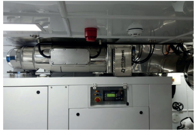
Even 400 mm was sufficient height to install a DPF system.
