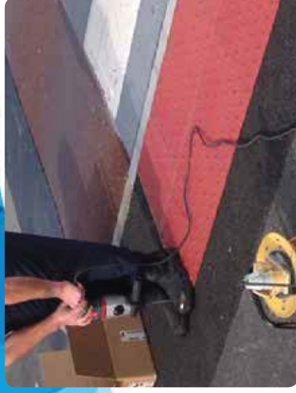
Installation of RediFix tiles
