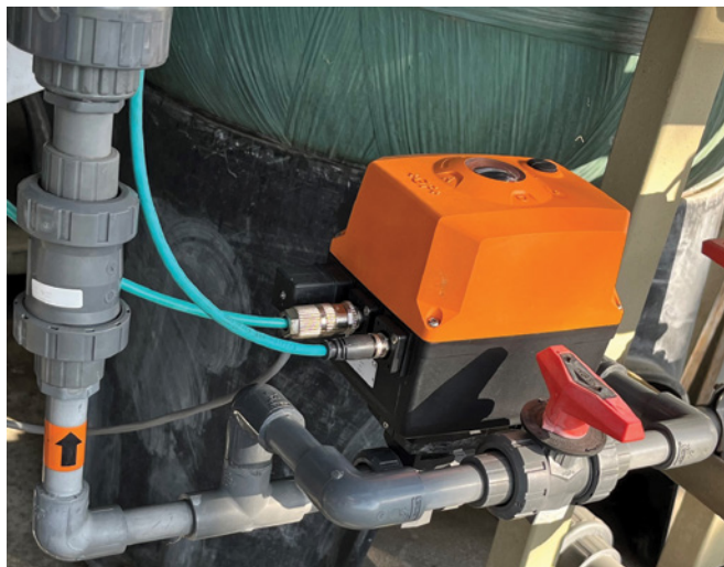
FIGURE 1. An automation upgrade using the EtherNet-equipped EA-25 electric actuator interface allowed an aerospace manufacturer to achieve greater efficiency for its onsite recycling process
