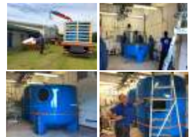
On site assembling
