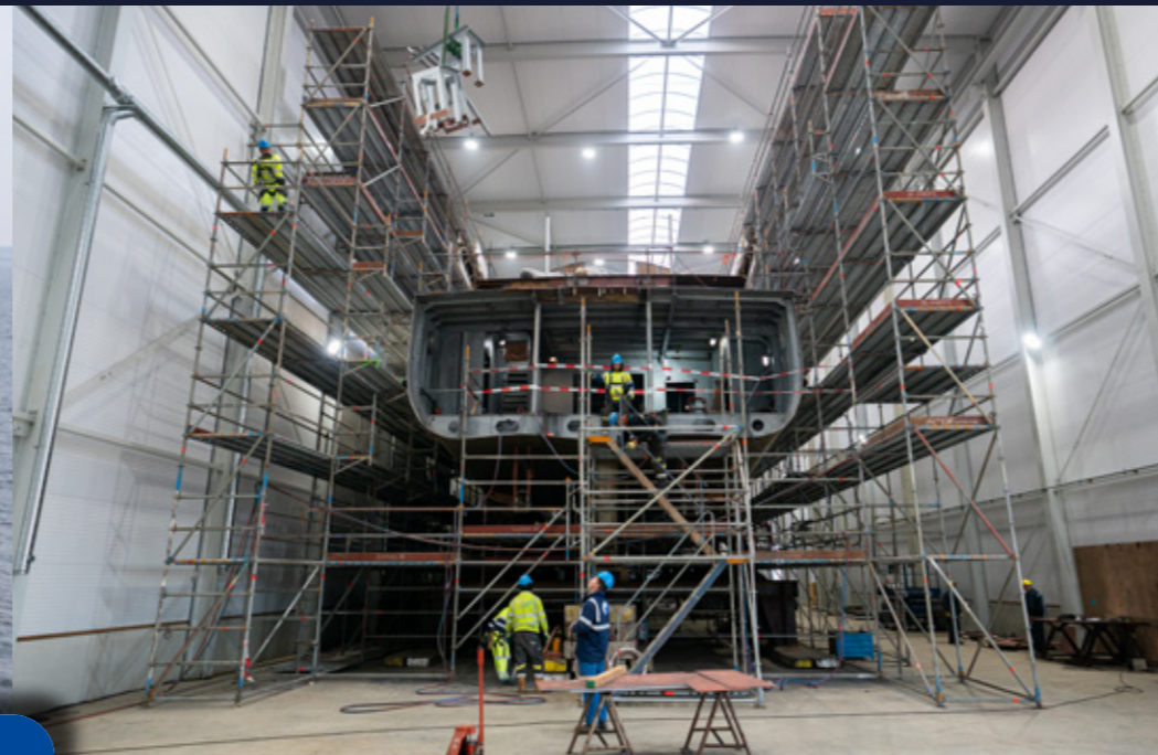
New covered yacht refit facility 70 x 20 x 18.5 m
