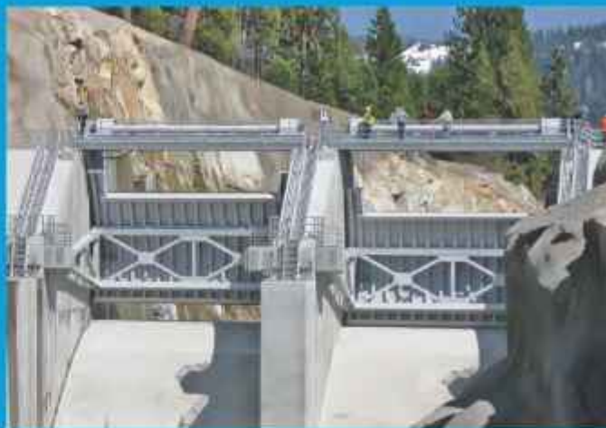
36.5' x 18.85' Tainter Gates L.L. Anderson Dam, CA
