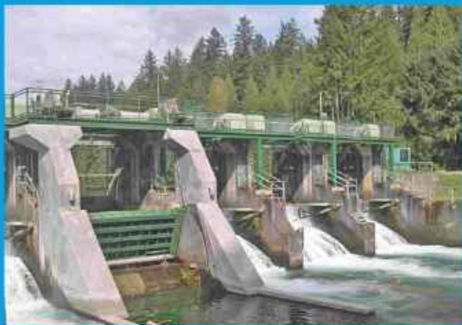
20' x 8', Crest Gates, Landsburg Fish Passage Ravensdale, WA
