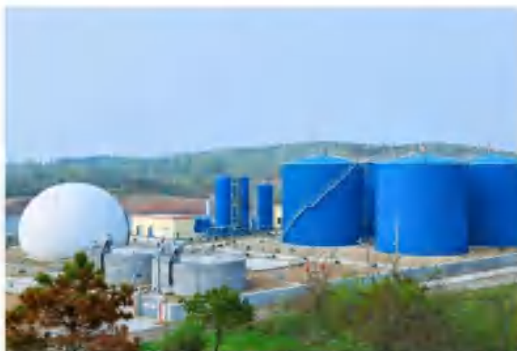
COFCO Wuhan Guangshui pig manure project
