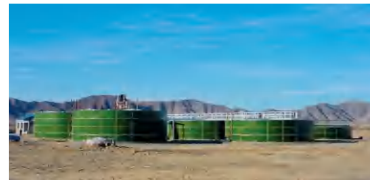
Jiuquan sewage project
