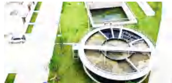
Urban sewage treatment integration AO project
