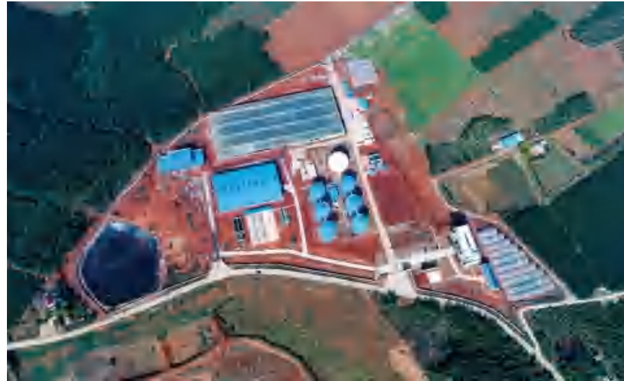
Xinyu centralized manure treatment plant
