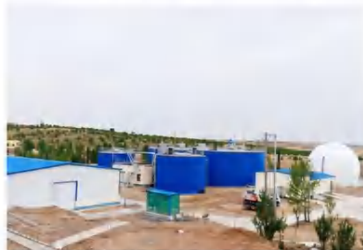
COFCO Chifeng pig farm project
