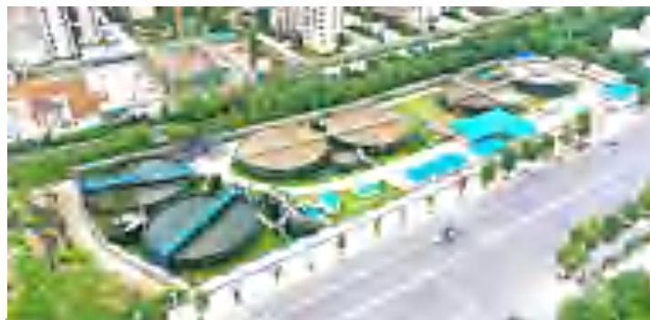
Guangxi Guilin sewage project
